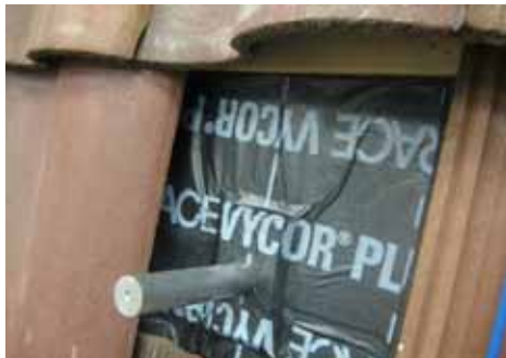
Universal Mount for Flat and Curved Tile Mounts. Fully water-proofed at sub roofing.
